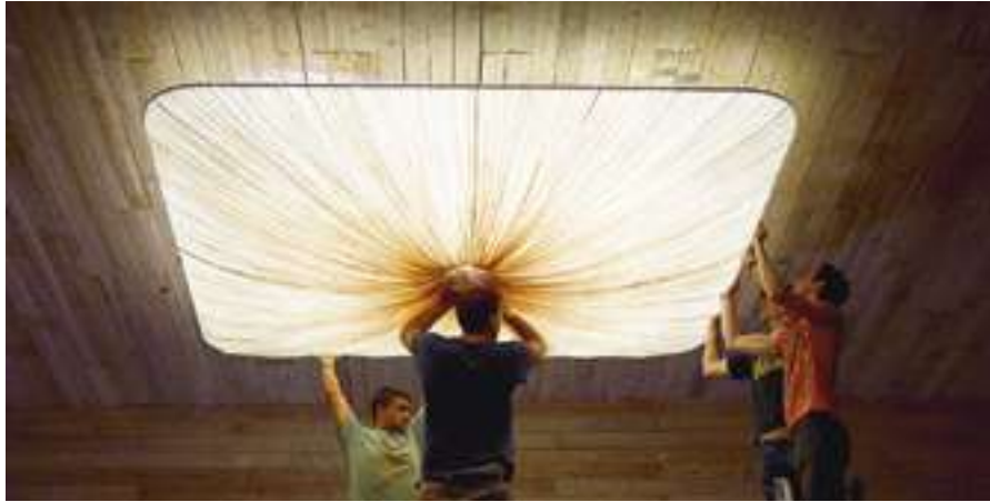
Test installation of Custom Nara 240cm / 94"
